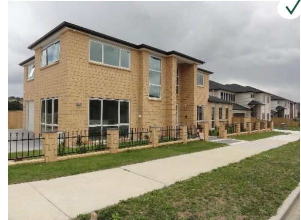
Fence for a corner section above is 3m back from the road boundary.
