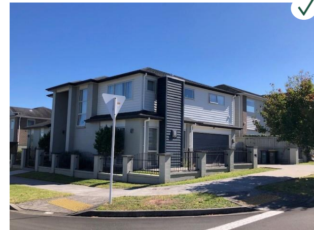
Fence for a corner section above is high quality and see through.
